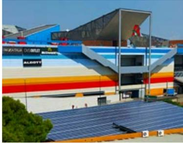
The Naples plant in Italy has a photovoltaic plant producing more than 630,000 kWh per year (approximately 10% of its electric needs), which brings a yearly saving of approximately 500 tons of CO<sub>2</sub>.
