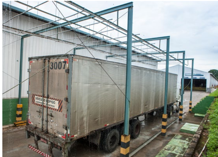
Rainwater reuse system in Manaus, Amazonas, Brazil, that is used to test water tightness on trucks
